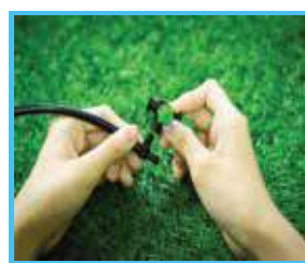
3. Connect the Fogger with T Coupling and measure the distance to put the Fogger.
